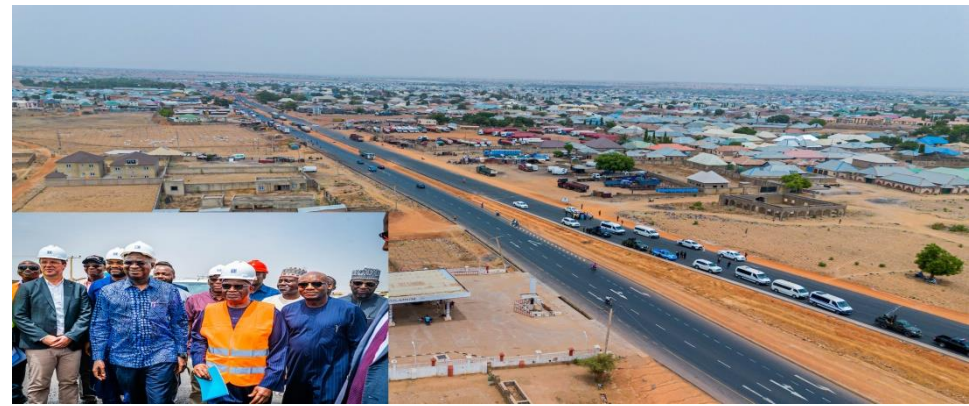
A view of the Completed Section of the Reconstruction of Abuja - Kaduna- Zaria - Kano Dual Carriageway (Section III : Zaria - Kano) on Monday 17th April 2023. INSET: Chief of Staff to the President, Prof. Ibrahim Gambari (2nd right), Hon. Minister of Works and Housing, Mr Babatunde Fashola SAN (2nd left) , Senior Special Assistant to the President, Special Projects, Mr Aniefiok Johnson ( right) , Managing Director, Julius Berger Nig Ltd, Mr Lars Richter (left) and others during the inspection of the Completed Section of the Reconstruction of the Abuja - Kaduna- Zaria - Kano Dual Carriageway (Section III : Zaria - Kano) on Monday 17th April 2023
