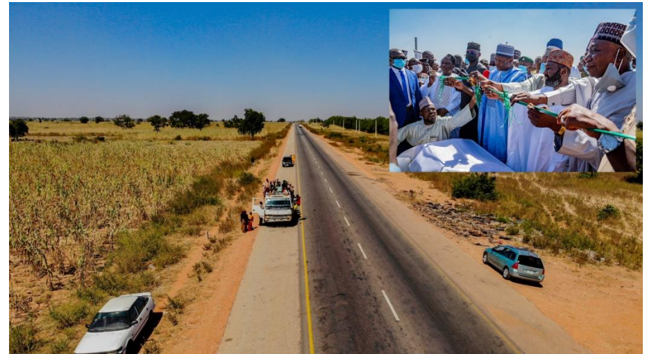
A view of the Sokoto - Tambuwal -Jega - Kontagora - Makera Road Phase I & II in Sokoto and Kebbi States during its Commissioning and Handover on Thursday, 25th November 2021. INSET: Representative of the President and Hon. Minister of Justice and Attorney - General of the Federation, Mr Abubakar Malami, SAN (2nd Left), Hon. Minister of Works and Housing, Mr Babatunde Fashola, SAN (left), Governor of Kebbi State, Mr. Abubakar Atiku Bagudu (middle)
