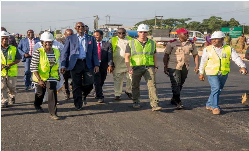
Hon. Minister of Power, Works & Housing, Mr Babatunde Fashola, SAN(2nd left), Federal Controller of Works, Ogun State, Engr. Joshua Popoola (4th right;behind), a Supervisor in the Ministry, during the Hon.Minister's inspection of the ongoing Rehabilitation, Reconstruction and Expansion of the Lagos -Ibadan Expressway on Thursday, 25th October 2018.
