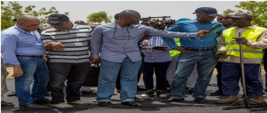
Hon. Minister of Power, Works & Housing, Mr Babatunde Fashola, SAN(2nd right) interacting with a Site Worker with Messrs. Mothercat Nigeria Limited, Mr Christopher Bulus (right). With them are Director Highways, Construction and Rehabilitation, Engr. Yemi Oguntominiyi(2nd left), Managing Director, Mothercat, Mr Jack El-Najjar (left) Director , Press in the Ministry, Mr Theo Ogeziachi (middle) and others during the Hon. Minister's inspection of the Rehabilitation of Hadejia -Nguru Road, Phase II - Kirikasama - Nguru in Jigawa State on Wednesday 9th May 2018.
