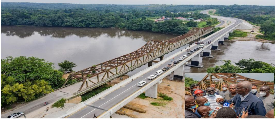
A view of the New Ikom Bridge built by the administration of President Muhammadu Buhari during an inspection visit by the Hon. Minister of Works and Housing, Mr. Babatunde Fashola, SAN on Monday 26th July 2021. On the left is the old Steel truss Bridge built 50 years ago in 1971. INSET: The Hon. Minister of Works & Housing, Mr. Babatunde Fashola, SAN(right) speaking with journalists shortly after the inspection of the New Ikom Bridge in Ikom, Cross River State on Monday, 26th July 2021.
